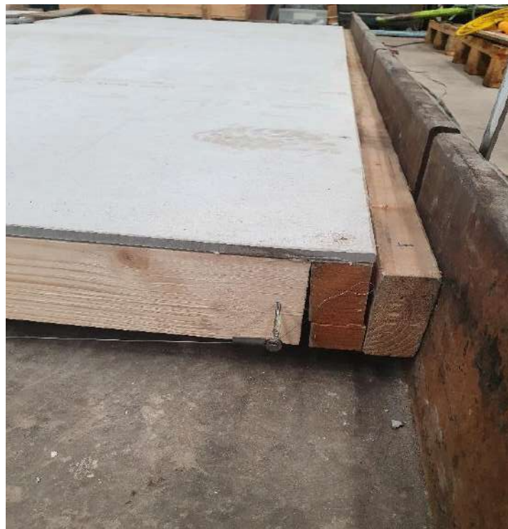
Plate 2 – Typical Mode of Failure
